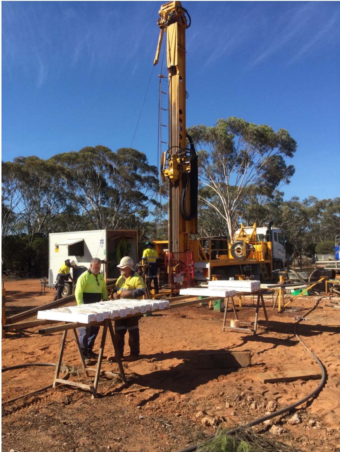
Figure 1: 14 March 2017 – Diamond Drill Rig at Lost Dog
